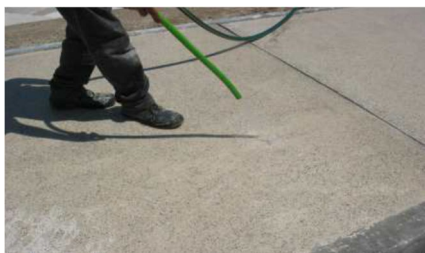
Cleaning the surface
