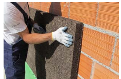
4. Fixing the panel by pressing it
