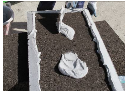
2. Applying ADHERE Vit ecoCORK on the back of the panels using the fixing method
