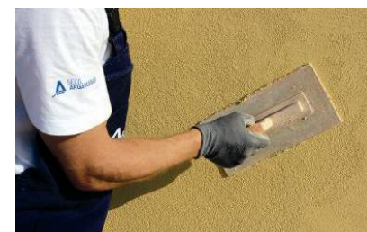
19. Application of acrylic finish REVDUR
