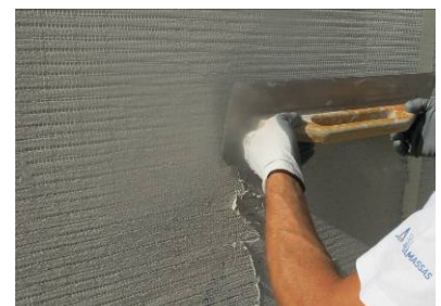
13. Second spreading of ADHERE Vit ecoCORK
