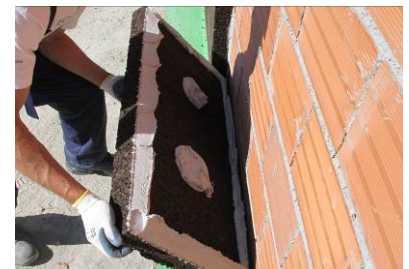
3. Placing the panel on the support
