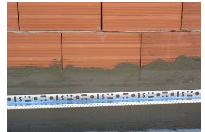
1. Fixing startup profile and support waterproofing.
