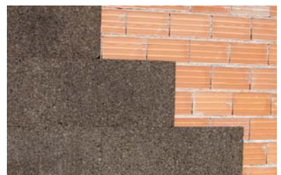
5. Placing the panels by rows
