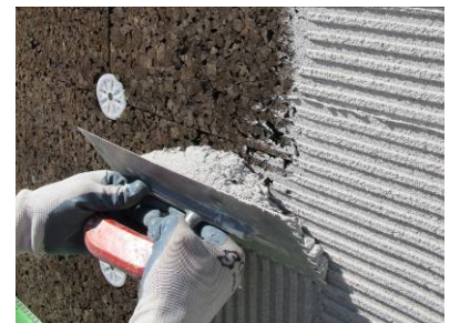
11. First spreading of ADHERE Vit ecoCORK
